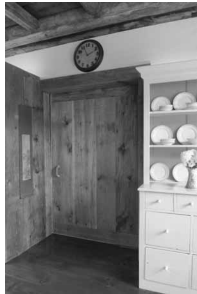
THE CLINCHED NAIL DOOR PROVIDES A QUIET BUFFER FROM KITCHEN NOISE TO THE DINNING AREA AND LIBRARY NOOK ON THE OPPOSITE SIDE.
