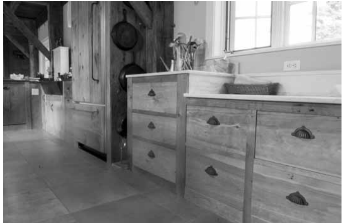
BULLARD USED A SINGLE PIECE OF WHITE PINE FOR THE FRONT PANELING OF THE DRAWERS — A SMALL TOUCH WITH HUGE ARTISTIC AFFECT.
