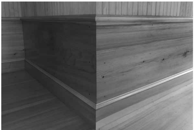
CONTRASTING GRAIN PATTERNS OF THE VARIOUS EWP TRIM ADD TO THE SHARP MODERNIST LOOK.
